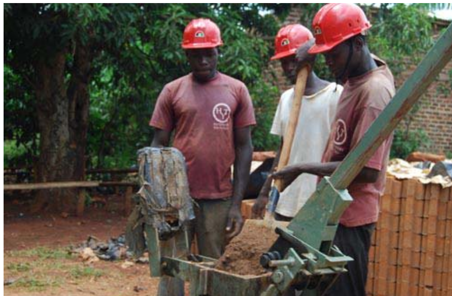
Figure 8: Filling the mould with soil/cement mixture.
