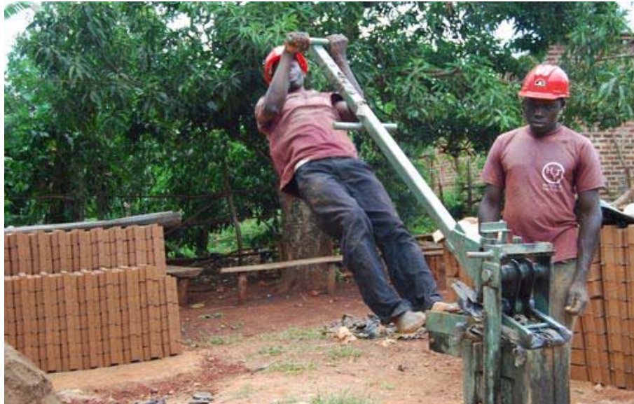
Figure 10: Worker bringing down the handle of a compacting machine.
