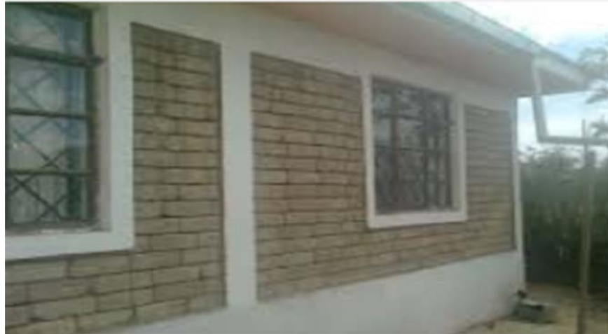
Figure 16: Protection around the base and corners with plastering.
