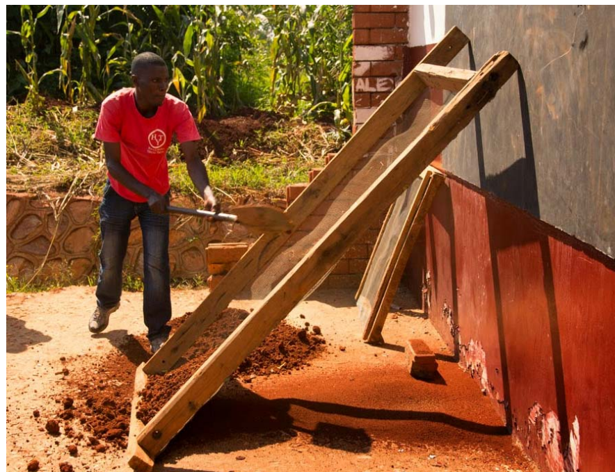
Figure 7: Sieving the soil with a wire mesh screen.
