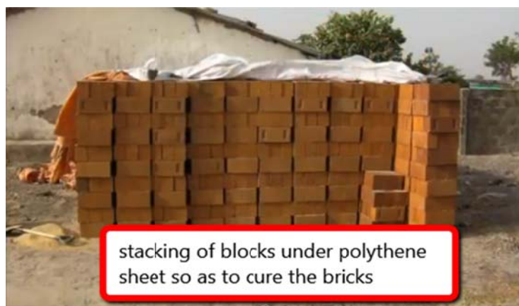
Figure 13: Blocks covered with polythene sheets.
