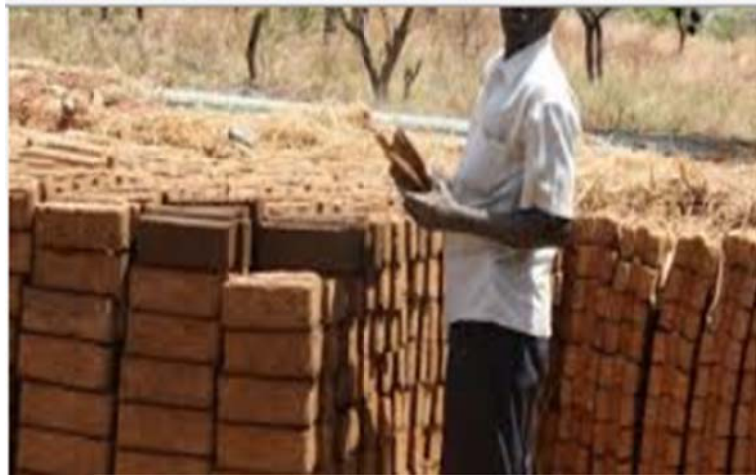
Figure 12: Curing blocks covered with grass
