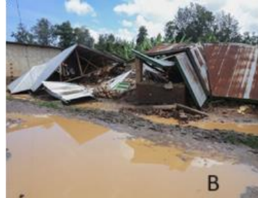
Figure 6: Photo showing the effects of a severe storm.
